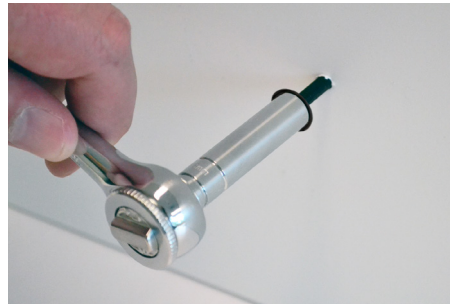
19b Below the counter, use a 8mm deepwell socket to tighten the 4 nuts.
